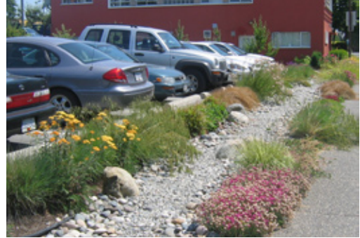
Stormwater management functions are integrated into the design of the parking field.
