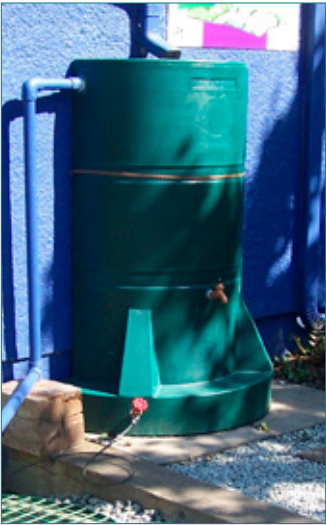
Rain barrels help capture rainwater for harvesting.
