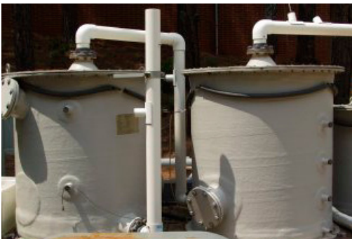
Bio filters for wastewater treatment are appropriate for use in residential buildings.
