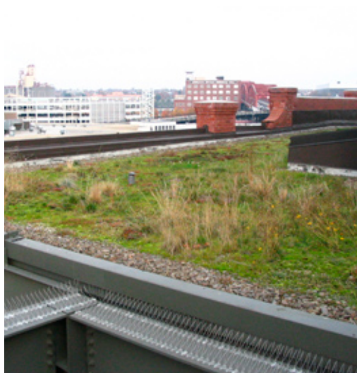
Green roofs help manage stormwater run-off at the building scale.
