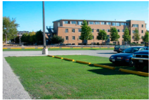
Permeable surfaces can be integrated into parking lots.
