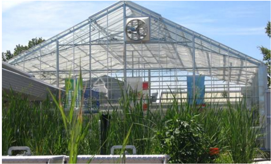
Solar aquatic systems transform wastewater solids into an organic soil amender.
