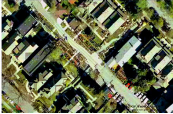
Figure 1: Garden Block - Mole Hill, Vancouver. This multi-unit mixed-use block includes a lane, parking, a cross-block greenway, and community garden plots.
