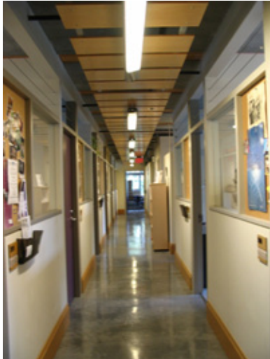
Figure 2: To reduce finishing materials, highly polished concrete flooring was used at the Liu Centre on the UBC campus.
